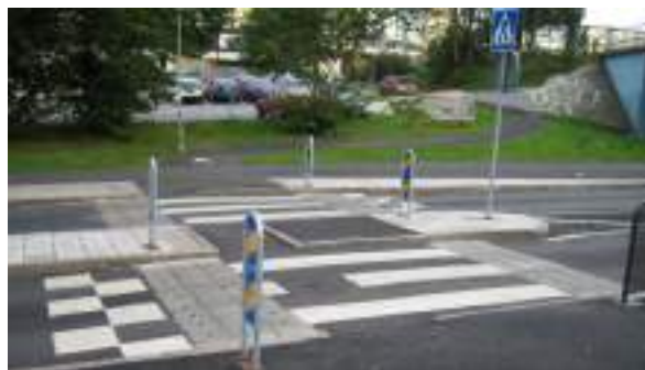
Figure 116: Improvement of adjacent pedestrian crossing and walkways and elimination of small obstacles on the pathways (Source: Landskapsgruppen AB, Emma Johansson eller Roland Ahlgren där ej annat anges)
