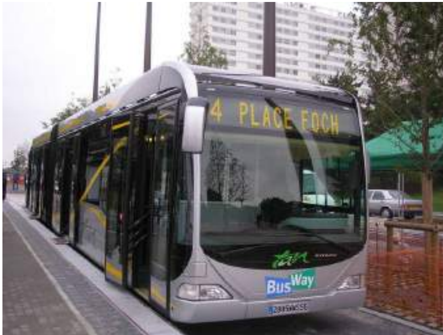
Figure 21: Nantes Busway: ramps (Source: https://tc-infos.fr/dossiers/bhns.php )
