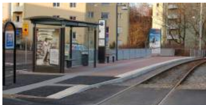
Figure 114: Higher Platform for facilitating boarding and deboarding (Source: http://www.eltis.org/discover/case-studies/improving-accessibility-transport-goteborg-sweden )
